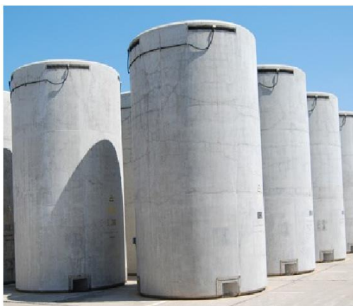
Fig 1. Storage containers for storage of spent nuclear fuel used on Zaporizhzhya NPP
